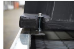
Fasten using carriage bolts
